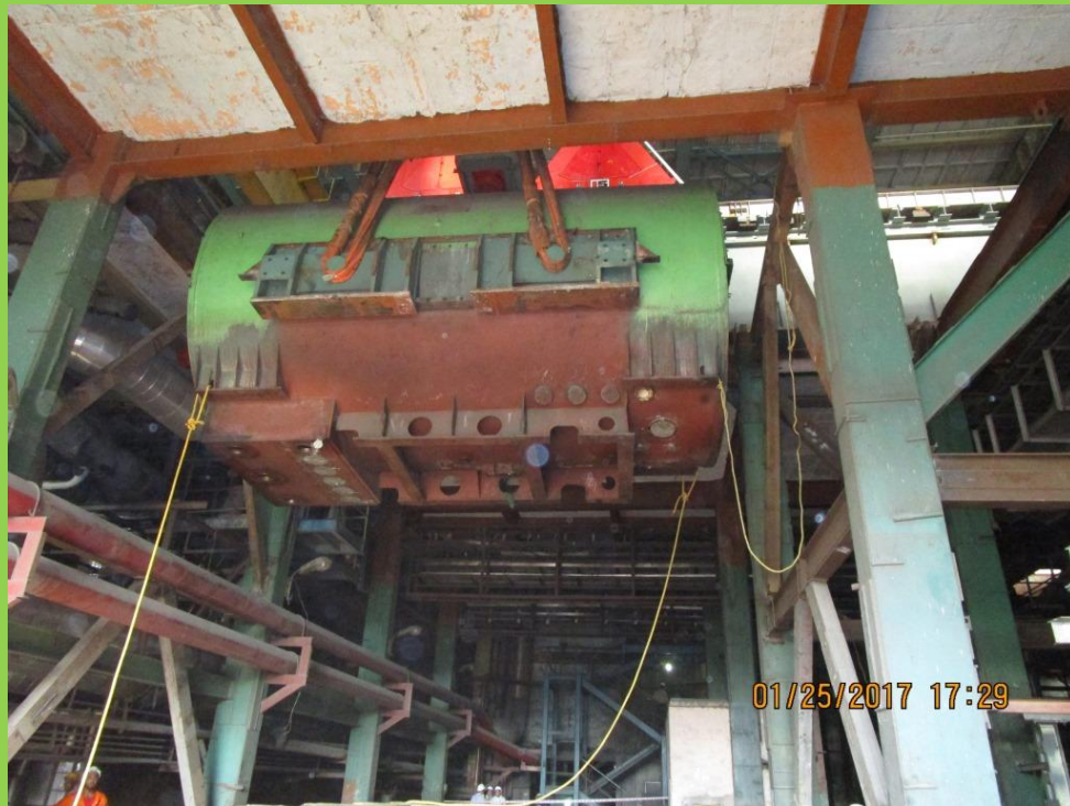
25-Jan-2017 - Old Generator Stator Unloading
