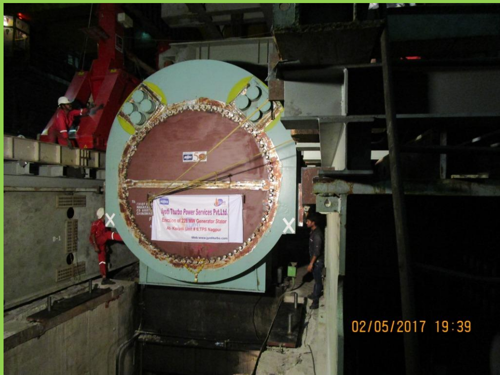
05-Feb-2017 - New Generator Stator Lifting & Shifting
